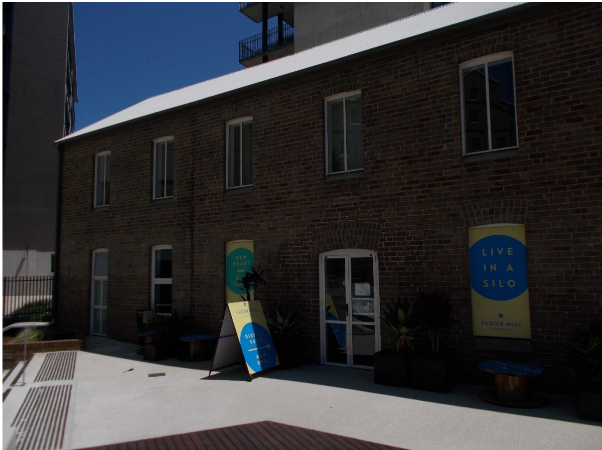
Photo 4 Site Photo with building 5E identified
