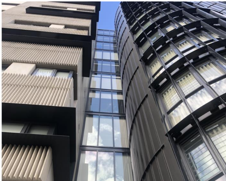
Photo 7 – Photo detailing existing hallway windows
